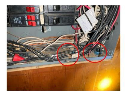
Subpanel 65: Wires are loose where it enters the subpanel. Recommend the cable be secured by installing an approved connector.
