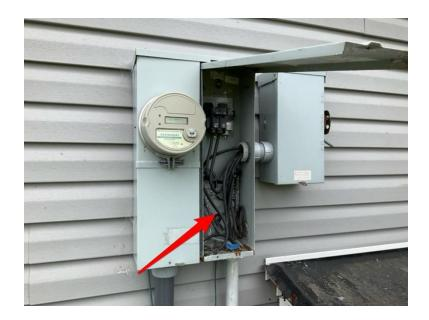
Subpanel 64: Wiring within the subpanel is not properly terminated.
